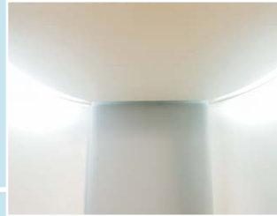
controllable dimmed ceiling downlighting
